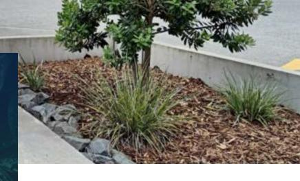
Biological treatment system that will remove the majority of contaminants, reduce stormwater flows and blend in to the urban environment.
