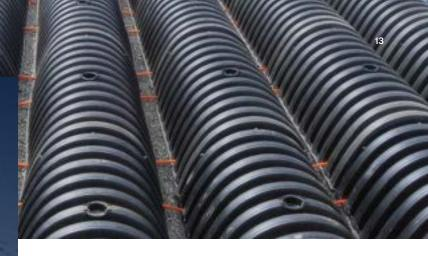
Stormwater chambers allow both retention and detention of stormwater so they can be used as either a traditional stormwater management tool or a green infrastructure device. In detention applications, the chambers can be sealed with an impermeable membrane to create an underground waterproof tank structure, and is ideal to maximise storage capacity in a shallow footprint.
