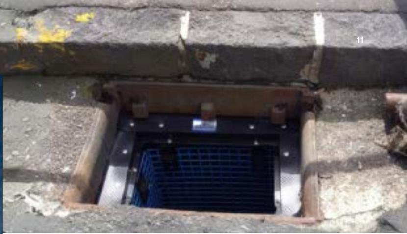
A low-cost solution that involves inserting a screening and sedimentation device into new or existing catchpits. Capturing pollutants at source allows hotspot targeting and can reduce maintenance costs for downstream stormwater treatment devices and infrastructure.
