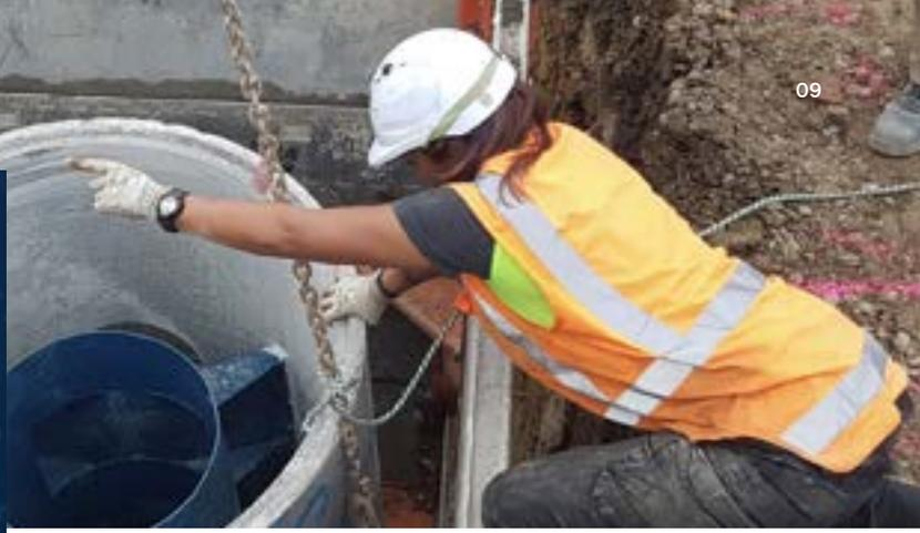
The Cascade Separator™ is the newest innovation in stormwater treatment. This innovative hydrodynamic separator excels at sediment capture and retention while also removing hydrocarbons, litter, and debris from stormwater runoff.
